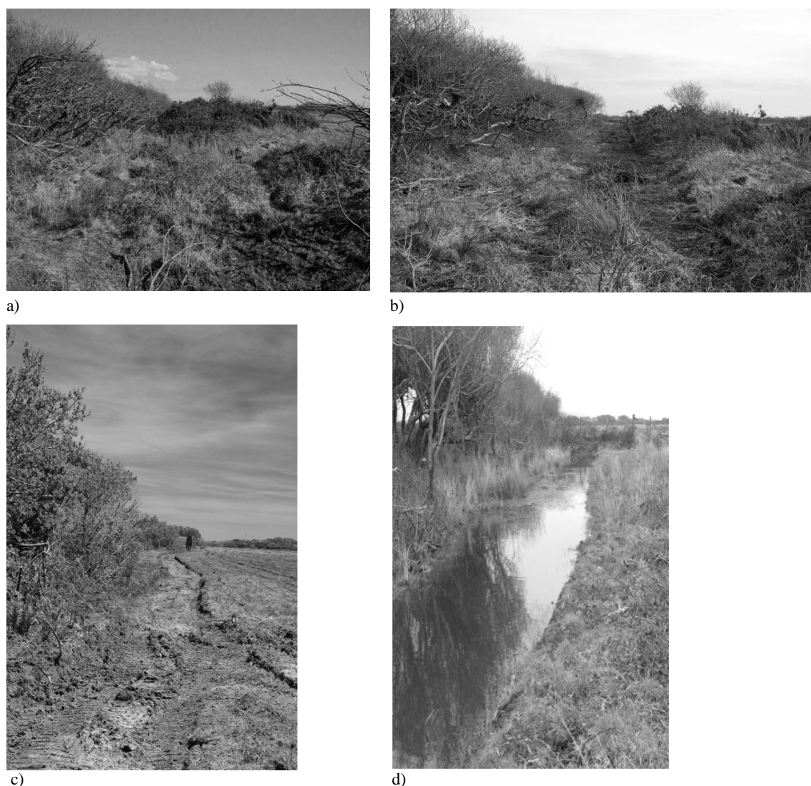
Figure 2: Sections of the northern track: a) overgrown before restoration work; b) after scrub clearance but before excavation; c) immediately after excavation in March 2010; and d) in late winter 2011 (photograph taken in February 2011 when the track was still inundated with water). The section shown in d) contained a single plant of Three-lobed Crowfoot in February 2011, and sizeable colonies of Pigmy Rush and Yellow Centaury when surveyed in late May 2011. (Photograph credits: a), b) and c), Andrew Pay; d) Amanda Scott.
