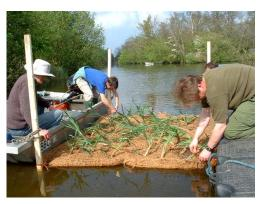
**Figure 1.** Installation of a coir pallet and planting of bulrush *Schoenoplectus lacustris* and reedmace *Typha latifolia*.
