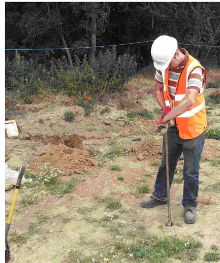
**Figure 2.** Hand-augering to locate tunnels and chambers along the line of the water main. The exposed badger tunnels can be seen emerging from the base of the hedge, one has been fitted with a badger gate (left-hand edge centre of photograph).
