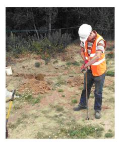
**Figure 2.** Hand-augering to locate tunnels and chambers along the line of the water main. The exposed badger tunnels can be seen emerging from the base of the hedge, one has been fitted with a badger gate (left-hand edge centre of photograph).
