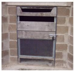
**Figure 3.** Cave door made of steal and oak boards. The top has two slots for the bats to enter and exit the cave. The bottom is made of wire mesh to enhance ventilation.
